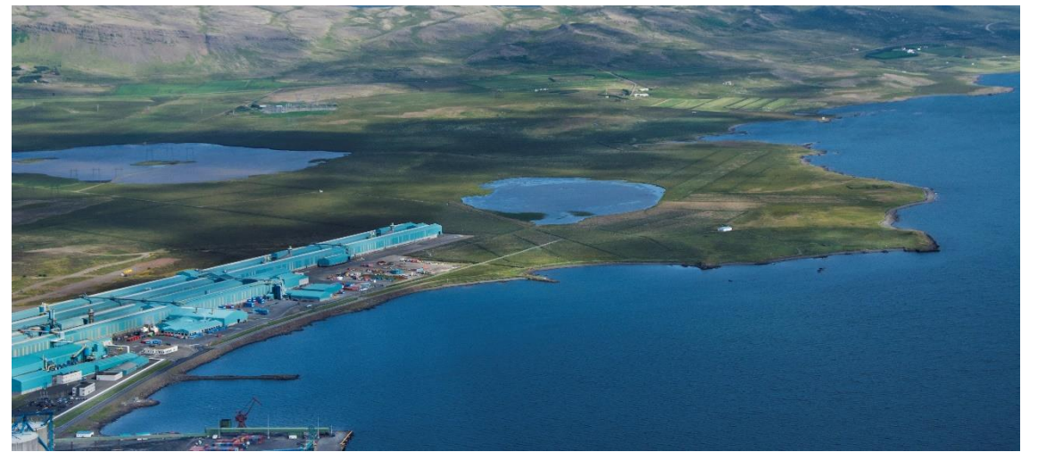
Aerial view from the west with Grundartangi Harbour in the foreground.
