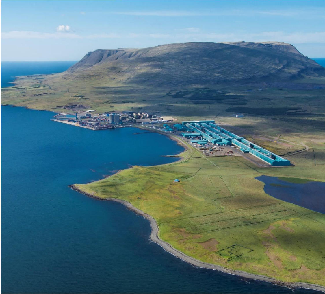
Aerial view from the east with project location in the foreground.
